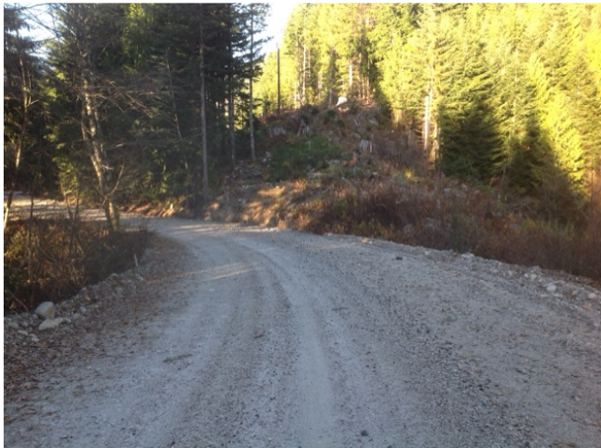
Approach from Left Bank when facing downstream
